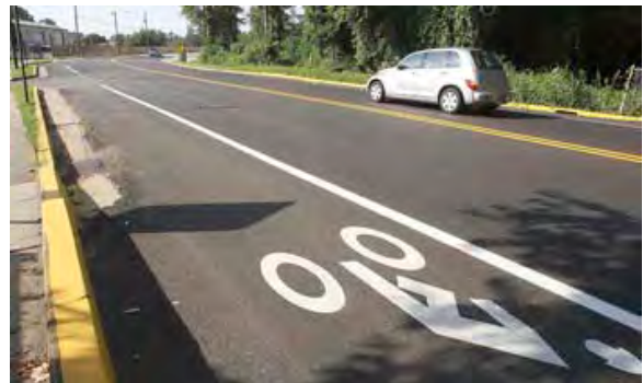
Figure 12 Bike lanes recently installed on Sustella Avenue in Valdosta. Source: Valdosta Daily Times
