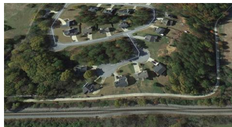
Figure 8 Silver Comet Trail near Rockmart, GA (Source: Google Earth)
