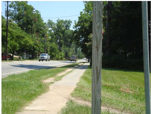
Along Goodman St., between Patterson St. and Alabama St., there are sidewalks located along both sides of the road. The sidewalks are in good shape, appear to be well-maintained, and they are separated from the roadway by a safe distance. There is little to no lighting provided along Goodman St. in Sparks, which is a concern for pedestrian safety. There are also few marked crosswalks for pedestrians to use, and
