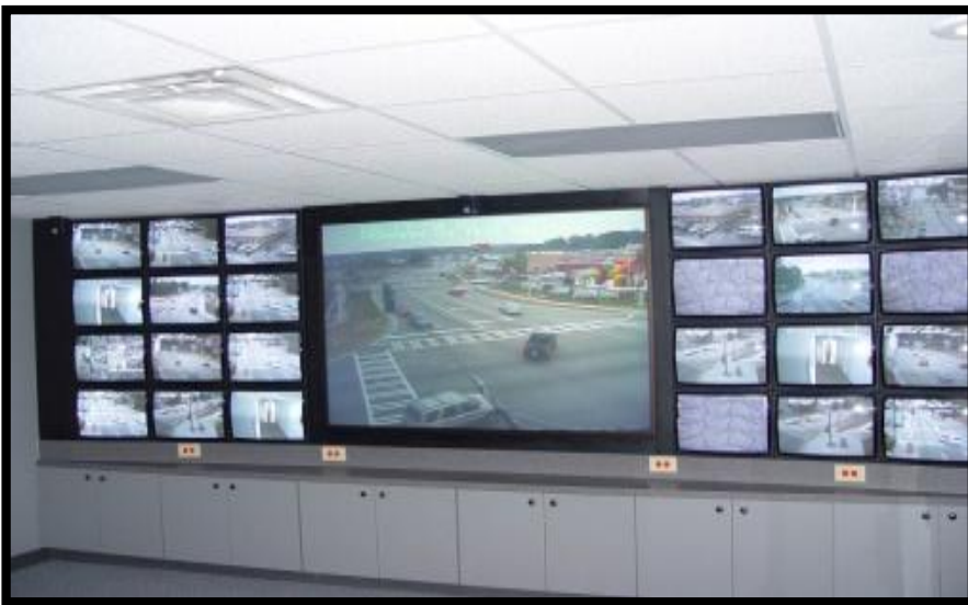
*Traffic Management Center
