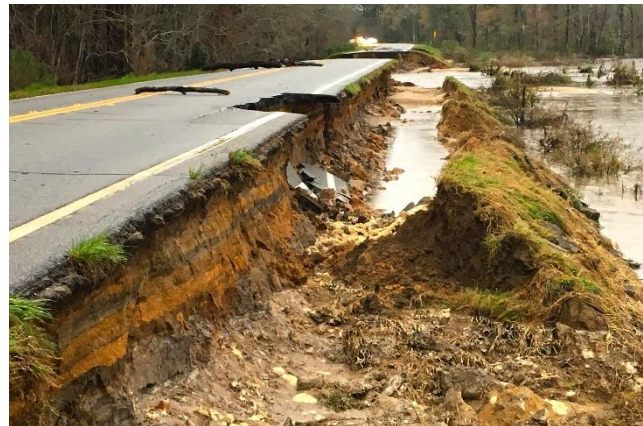
FIGURE 14: SR 112 IN WILCOX COUNTY, GA WASHED OUT DUE TO HEAVY PRECIPITATION IN MARCH 2020 SOURCE: GDOT
