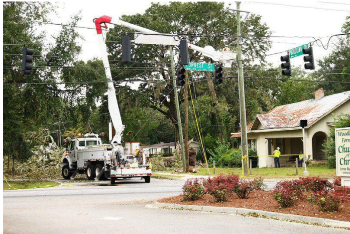
FIGURE 5: CREWS CLEAR DOWNED TREES FOLLOWING HURRICANE IRMA IN SEPTEMBER 2017
