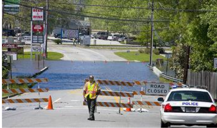
FIGURE 3: WATER OVERTOPPING ALONG GORNTO ROAD AT SUGAR CREEK DURING APRIL 2009 FLOODING EVENT SOURCE: VALDOSTA DAILY TIMES
