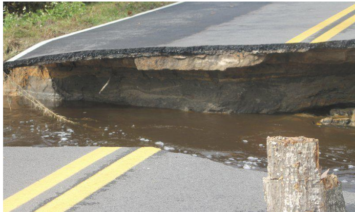
FIGURE 4: PART OF OLD LAKE ROAD COLLAPSED DUE TO FLOOD WATERS IN DECEMBER 2018 SOURCE: VALDOSTA DAILY TIMES
