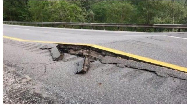
FIGURE 13: PORTION OF I-79 IN WEST VIRGINIA BUCKLED DUE TO EXTREME HEAT AND HUMIDITY IN 2018 SOURCE: WCHS (CHARLESTON, WV)
