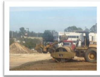
Figure 3 Construction of Gornto Road Extension in Valdosta
