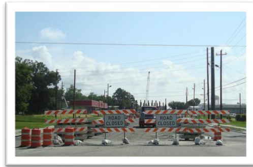
Figure 1 Construction of US 84/W Hill Avenue Overpass
